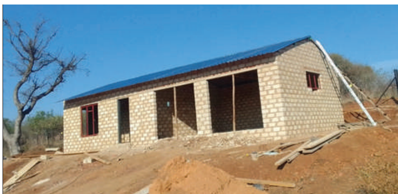
The farmhouse structure ready for plastering and finishes, 2023
