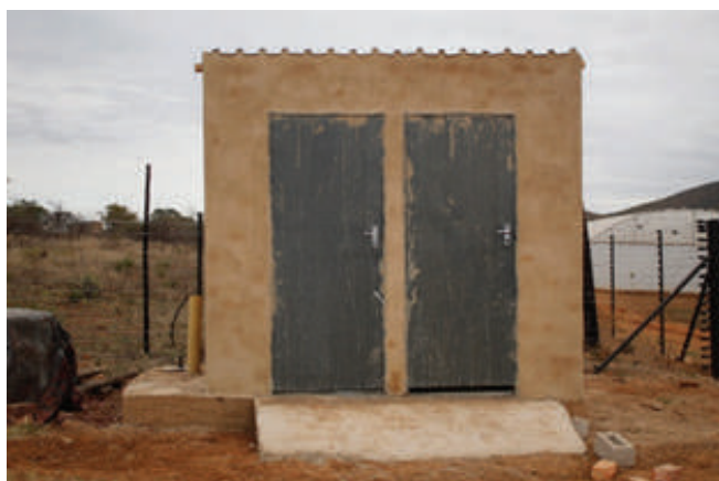
The hygiene centre toilet, 2023
